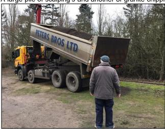
car park these should keep the crew busy at least to the start of the season. The scalping's will be used to bank the sides of the track where the ground is falling away and once the agreed level is obtained the granite chippings will be put on top of to the to further sleepers consolidate the track. An added bonus is that it also makes for a safe walkway for people
